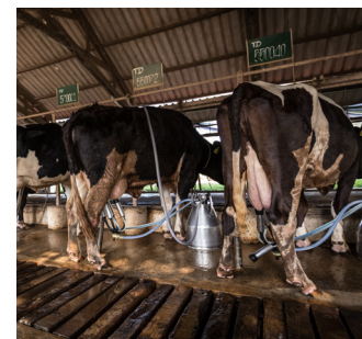
VFD on dairy milking, vacuum and transfer pumps
