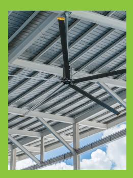
**Energy savings:** HVLS fans reduce the burden on HVAC systems by improving air circulation and enabling thermostat adjustments that can lower heating and cooling costs. With fewer high-speed fans needed, facilities may save energy and money
